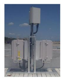
Cobham Wireless designed a system that used a base station hotel and optical master unit housed within existing telecoms infrastructure located 200m from the coastline. This was then connected to the remote units along the shoreline using fibre optic cables, ensuring it met the strict environmental laws in the region. The system is triple band: LTE 1800MHz, LTE 2600MHz and UMTS 2100MHz.
